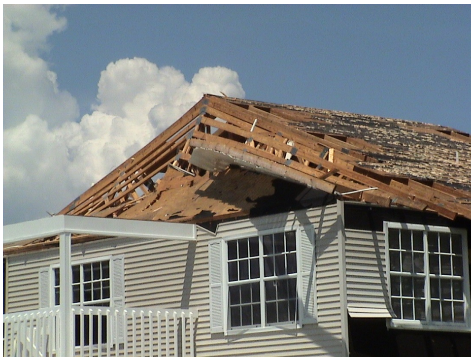
Figure 7. The most common gable end failure is one where the wall loses support along its top edge because sheathing is blown off. The wall may fold outward or be blown inward.
