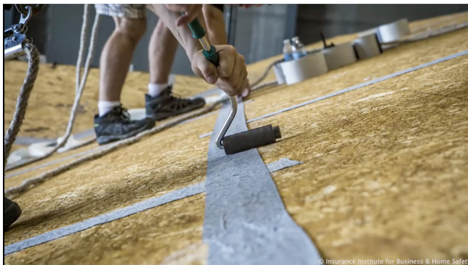
Figure 2-6. Installing a sealed roof deck system; taping the seams of roof sheathing.
