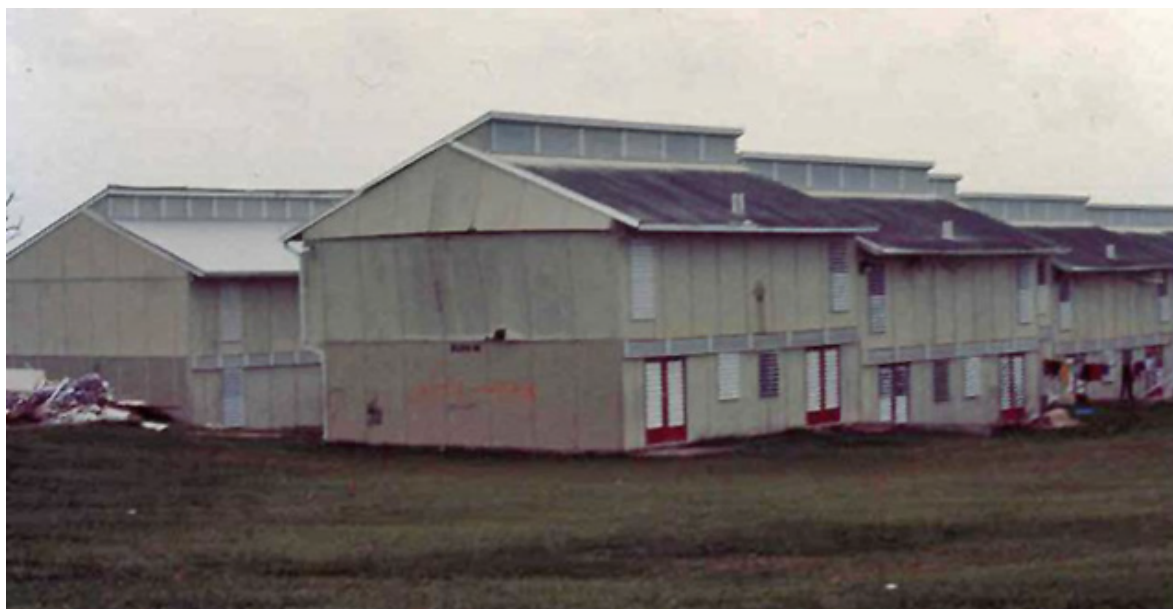
Figure 8. The second most common type of gable end failure is at the connection between the rectangular and triangular walls. Here the failure is just starting.
