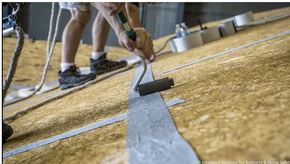
Figure 2-11. Installing a sealed roof deck system; taping the seams of roof sheathing.
