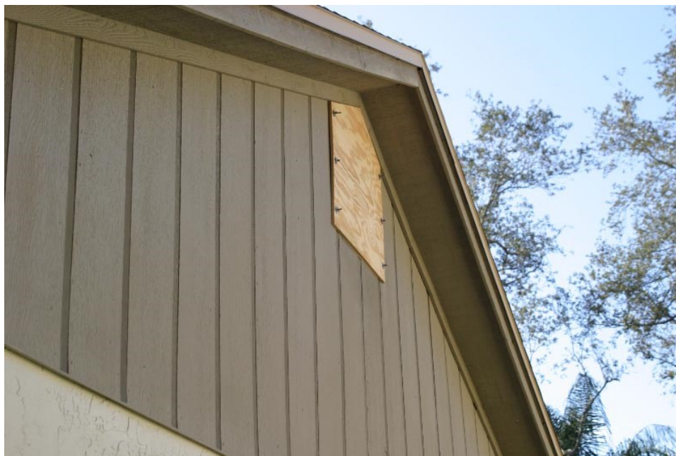
Figure 2-3. Outside covering of a gable end vent with plywood.
