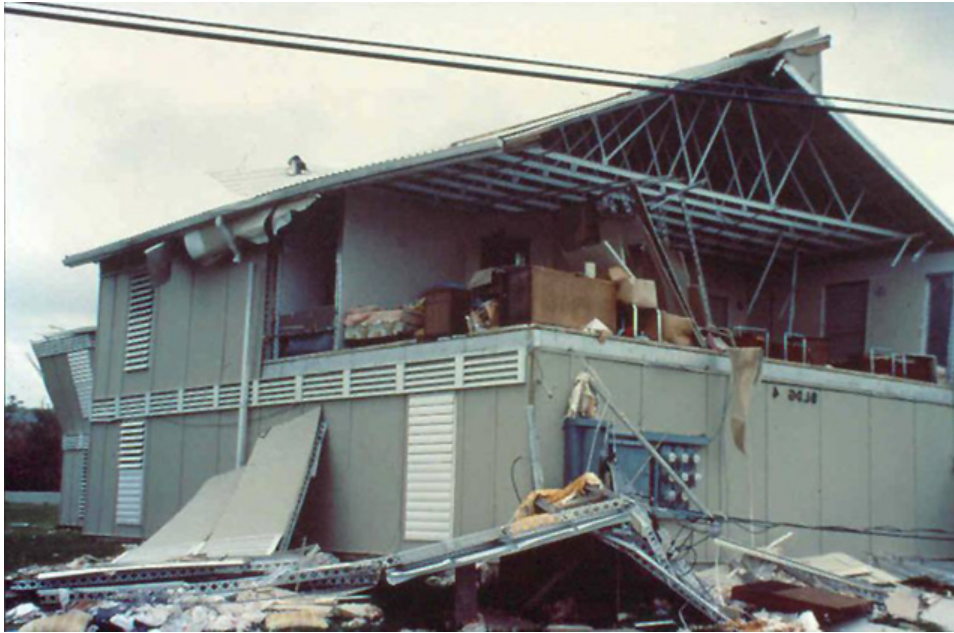
Figure 9. The more usual result of wall connection failures is a missing gable end wall and the wall below.
