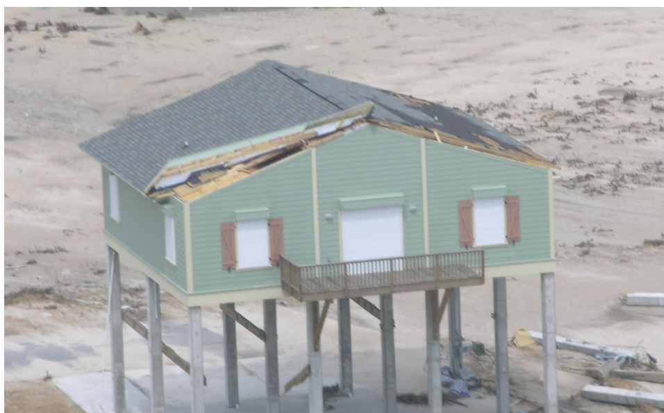
Figure 3-2. Gable end roof sheathing damage resulting from failure of outlooker connectors.
