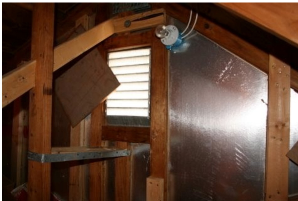
Figure 2-15. Gable end vent ready to be covered with plywood from inside attic.
