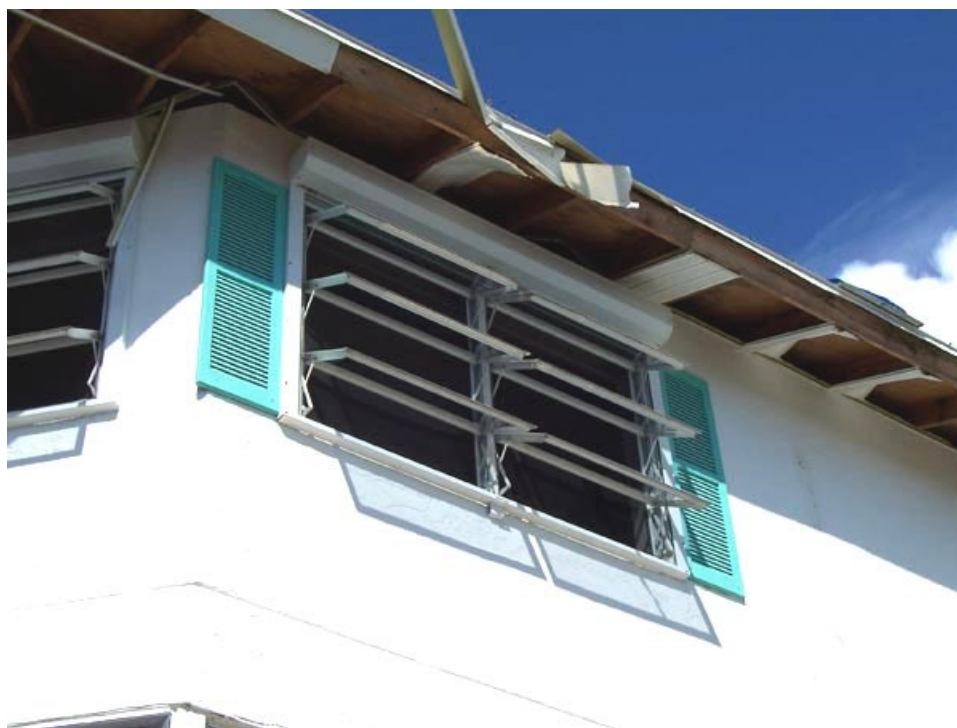
Figure 3-11. The loss of soffit material allows water to be blown into the attic.
