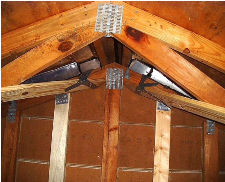
Figure 3-6. Blocking of gable rake soffit vents using metal flashing.
