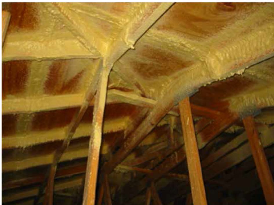
Figure 2- 1. Closed-cell polyurethane foam adhesive applied to the underside of the roof sheathing at the joints between the sheathing panels and along all intersections between roof sheathing and all roof framing members.
