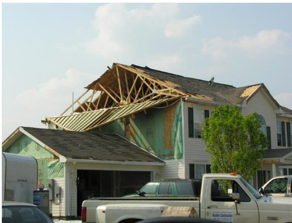
Figure 3-1. A gable end failure where the wall lost support along its top edge and is folded outward.
