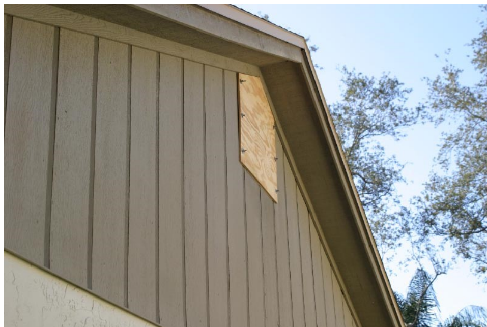
Figure 2-14. Outside covering of a gable end vent with plywood.
