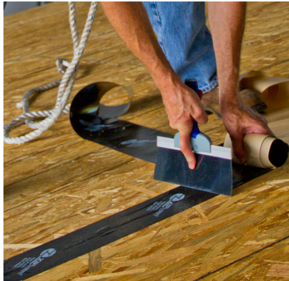
Figure 0-2. Applying qualified tape to roof deck seams using flat blade to eliminate voids and wrinkles.
