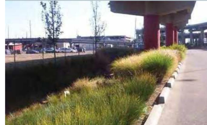
Bio-swale use in Parking Lots to Filter Pollutants from Stormwater Prior to Entering Sewer System
