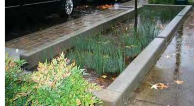
Green street techniques to filter stormwater before entering storm sewer system
