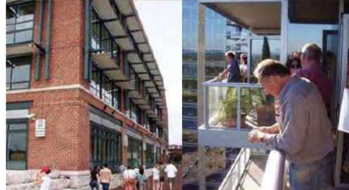
Cantilevered sun shades on windows to take advantage of natural lighting while regulating passive solar heating
